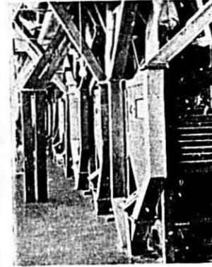
One line of purifiers at Capital "B" Mill
